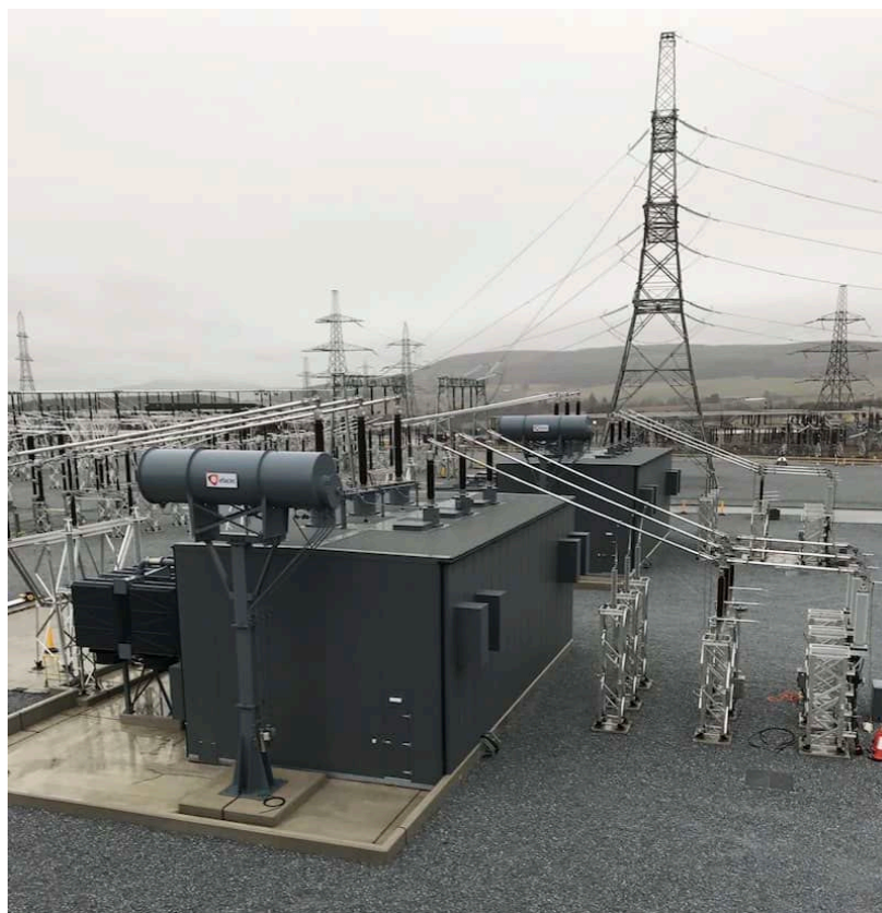
31. Figure 2: HVAC Transformer with -20dB Acoustic Enclosure. Credit: Siemens and Kimpton Acoustics Ltd
